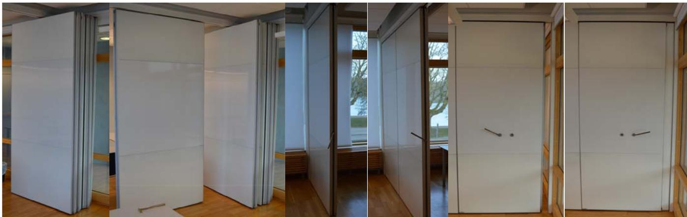
When setting up the partition, turn the folding section up so that it lines up with the ceiling rail, with the groove pointing towards its recess. It can then be slid along the rail towards the wall and locked with the handle into the lock recess in the groove. The last section is then turned up and both lock recesses are locked.
